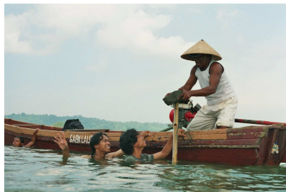
(c) Tide gauge installation in Seleko.
